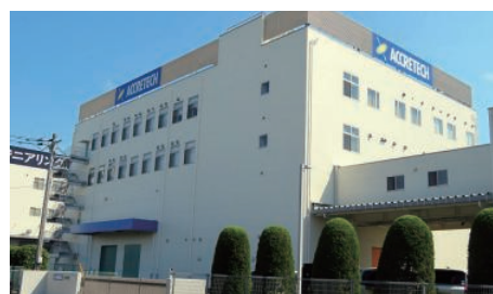
Tsuchiura Plant MI Building
