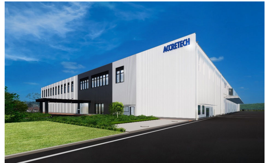
Nagoya Plant (Aichi, Japan) Operation scheduled for FY2025 Grinder-centered production system
